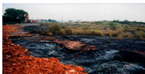
View of the lagoon at the beginning of the operation
