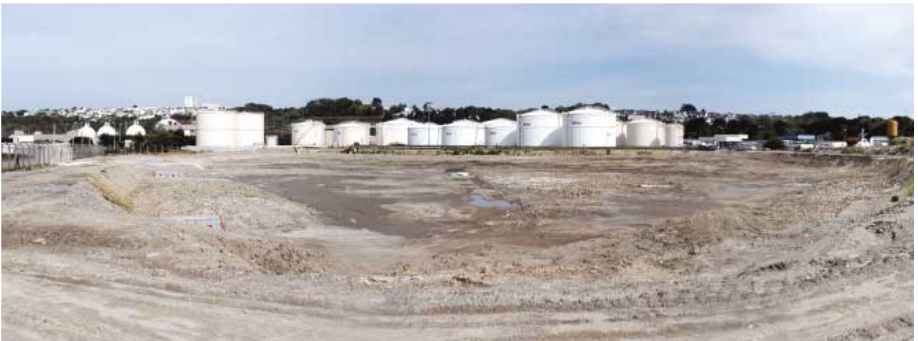
View of site after completion
