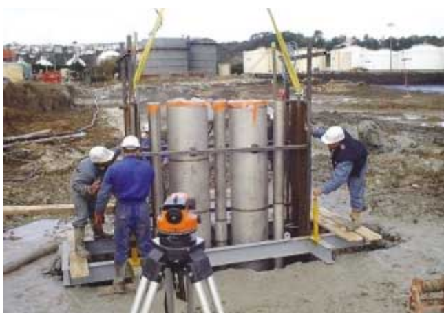
Installing filter gate
